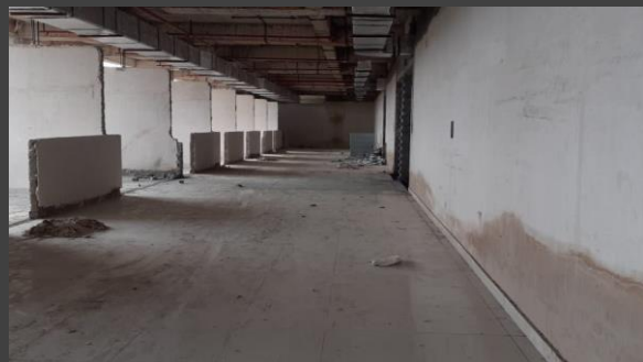
99C: Interiors; Work in Progress
