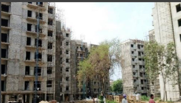
AP Flats: Work in Progress
