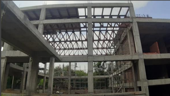
Sports Complex: Work in Progress
