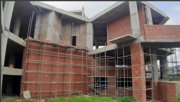
Sports Complex: Work in Progress
