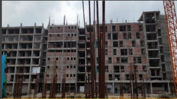
Boys' Hostel: Work in Progress
