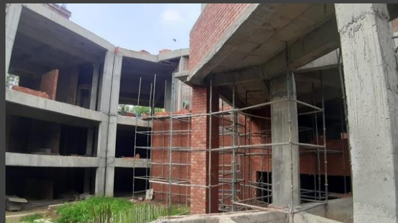
Sports Complex: Work in Progress
