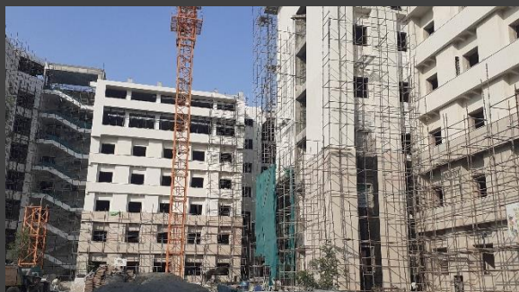
99B: Exteriors; Work in Progress
