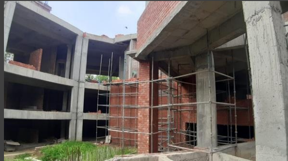
Sports Complex: Work in Progress
