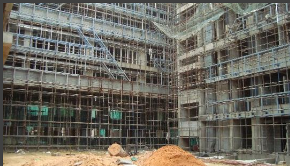
R & I Park: Exteriors; Work in Progress
