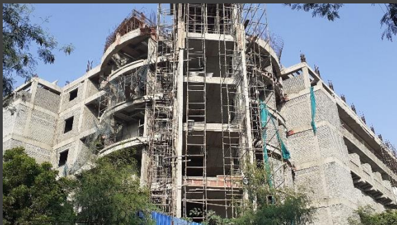
99C: Exteriors; Work in Progress
