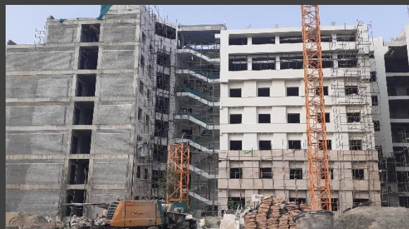
99B: Exteriors; Work in Progress
