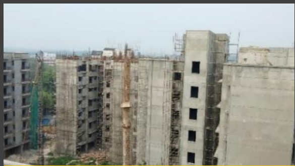
AP Flats: Work in Progress
