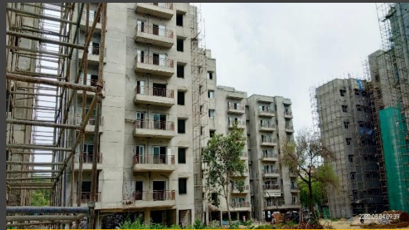
AP Flats: Work in Progress
