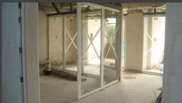
R & I Park: Interiors; Work in Progress
