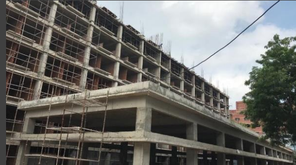
Girls' Hostel: Work in Progress
