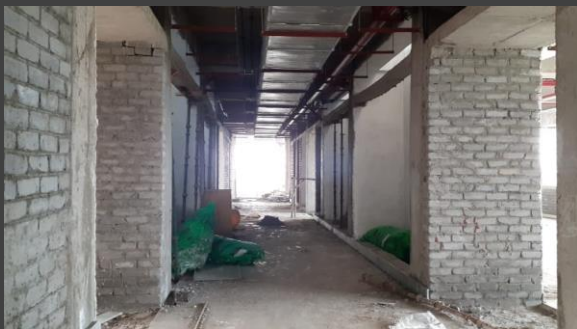
99C: Interiors; Work in Progress
