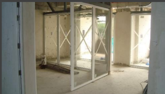
R & I Park: Interiors; Work in Progress
