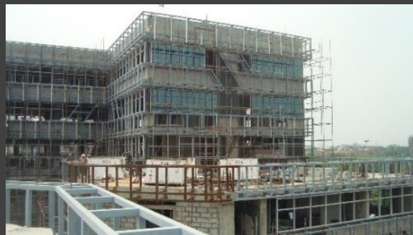
R & I Park: Exteriors; Work in Progress
